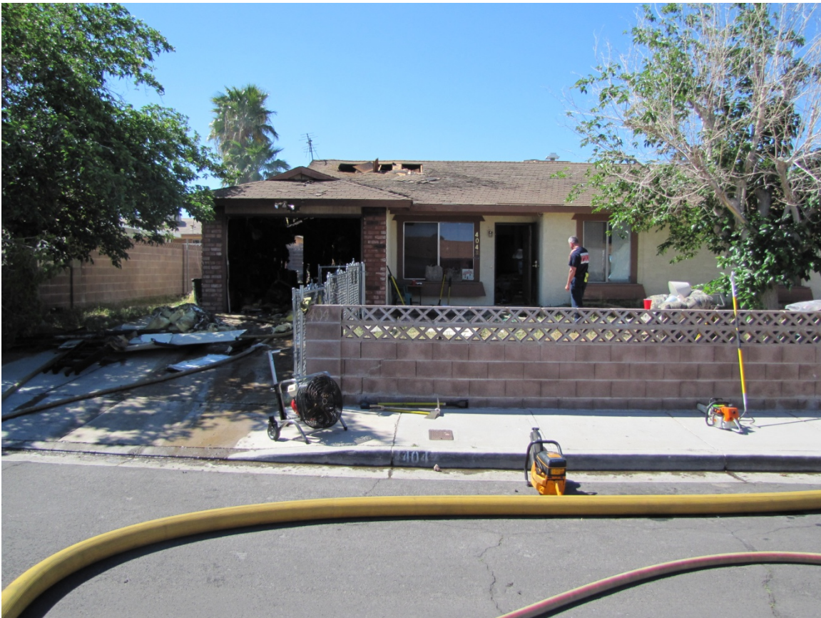
Figure 1: A side of structure showing garage and ventilation holes.
